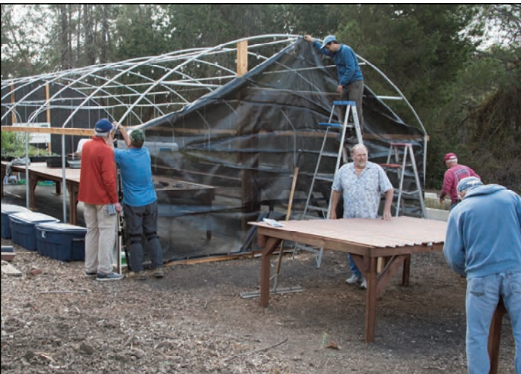
Left: Volunteers install shade cloth and build hardening tables at the new CIR Camarillo nursery. Right: Completed nursery and hardening tables.
